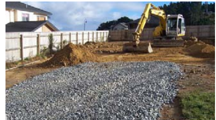
Figure 1 - Vehicle entry/exit pads (Source: www.pcc.govt.nz/ )
