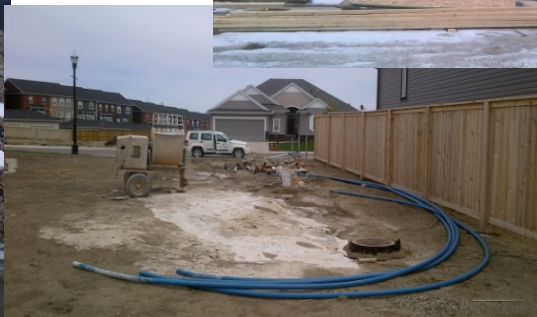
Concrete wash being dumped directly into storm system (above)
