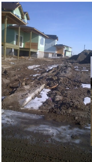
Concrete Drainage Swale covered in soil materials (left)
